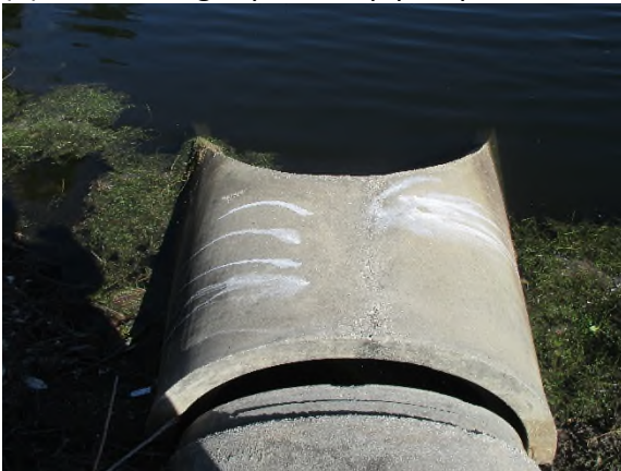
(9) Crack along top of the pipe tip
