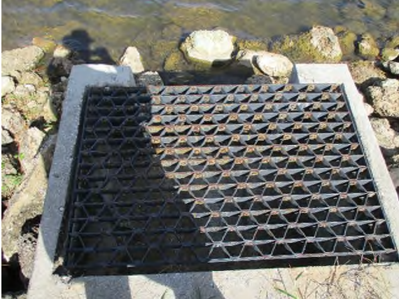
(3) Control Structure not flowing
