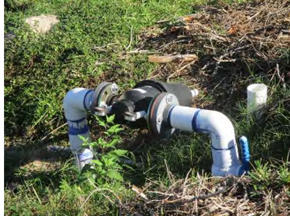
(4) Unburied line leading out into lake
